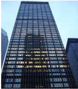
JPMorgan Chase Headquarters 270 Park Avenue
