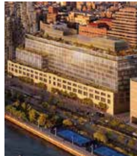
St John's Terminal - South
