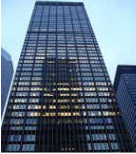
JPMorgan Chase Headquarters 270 Park Avenue
